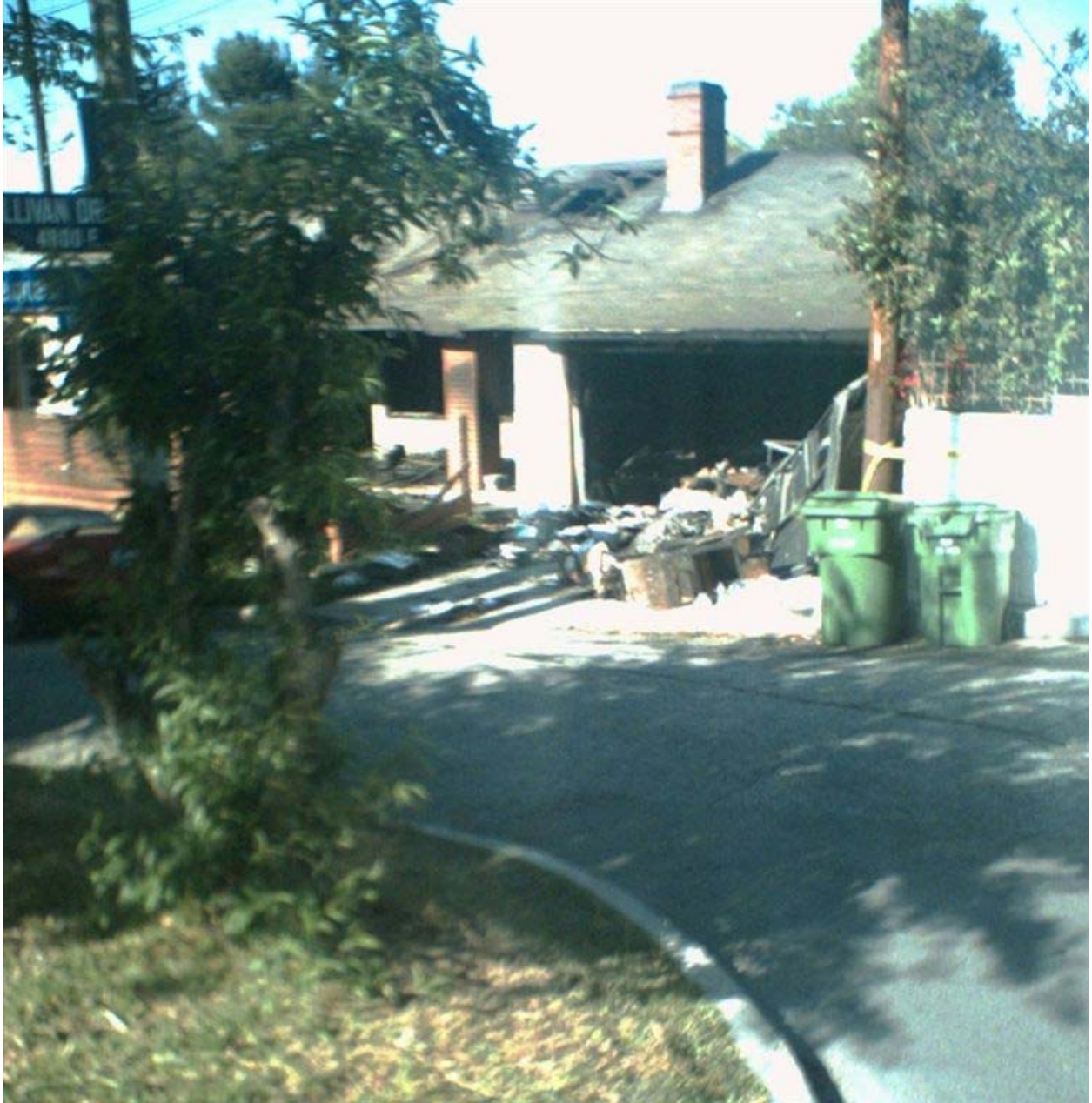
Gutted House where Two Dogs Freed by Firemen 04/19/2007
